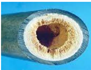
Figure 1. The scale corrosion on pipe
