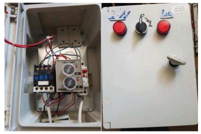
Figure (3.19). Electrical control system (Twin Timer)
