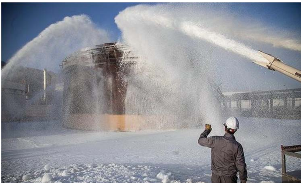
Figure 7.8 Storage tank fire operation using foam to suppress the fire.
