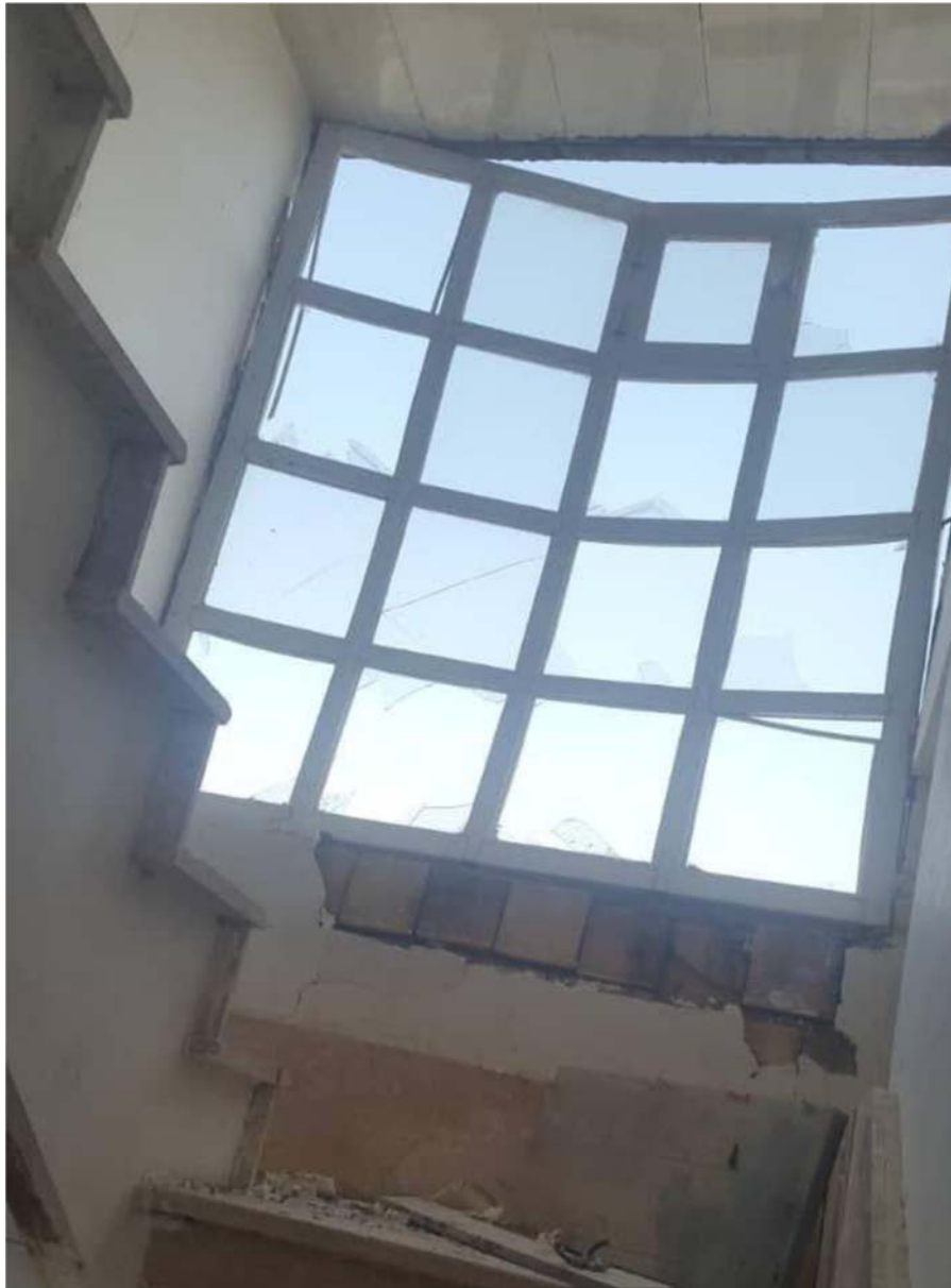
Figure 8.3 A semi-confined explosion due to natural gas leakage in a building.
