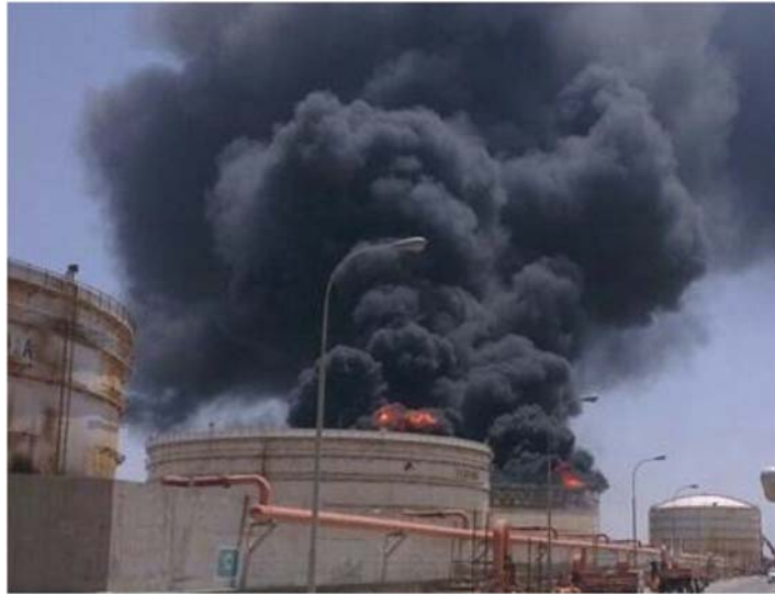
Figure 7.5 A large-scale tank pool fire.
