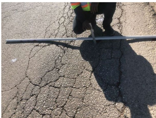
Fig. 2 Example to compute mean rut depth
