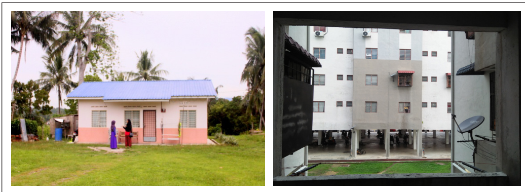
Figure 1. Single story, low-cost detached house with metal decking roof and plastered sand brick wall (Amir et al, 2019) (left), and high-density low-cost housing with air conditioning compressor on the facade (right)
