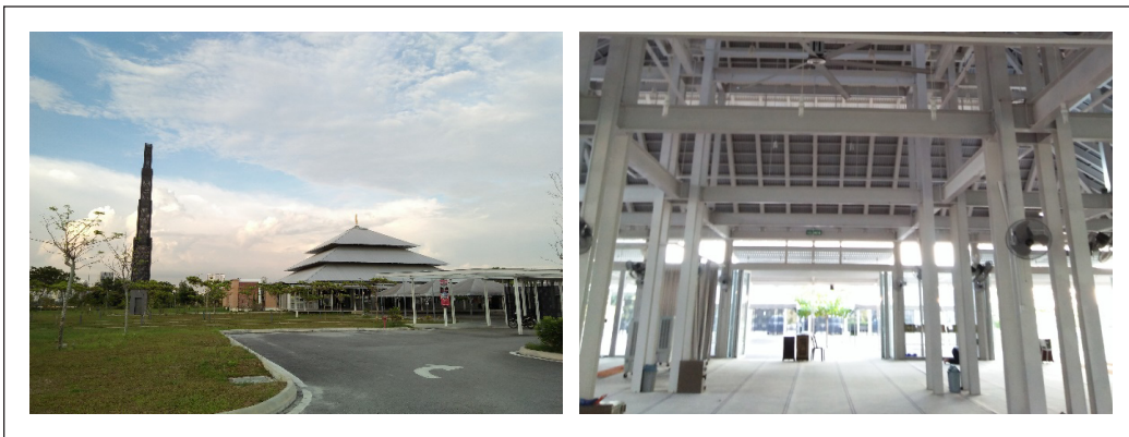
Figure 5. Modern mosque at Cyberjaya, Malaysia, has a large opening to optimise natural ventilation and lighting
