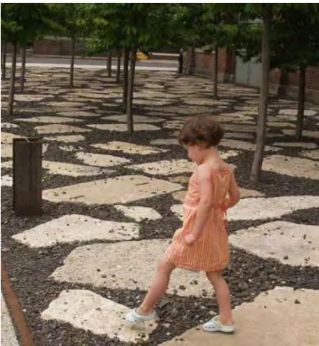
Fig. 7. A fragment of paving from recycled reinforced concrete panels. Source: D.I.R.T Studio, 2011
