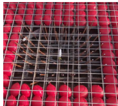
Fig. 5. Shear reinforcement.
