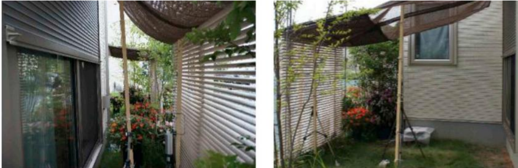
Figure(10): Evaporative cooling louver Source: [66]
