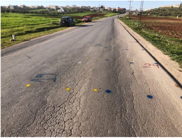
Fig. 2 Setting of grid on road surface
