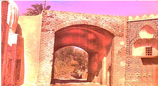
pl. 5. The vault mounted on arches of the gate
