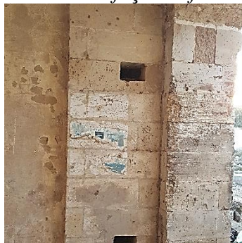
pl. 2. Inputs to place the latch that closes the wooden door of the gate inside
