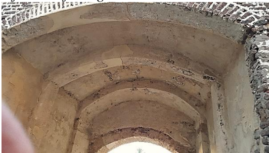
pl. 5. The vault mounted on arches of the gate
