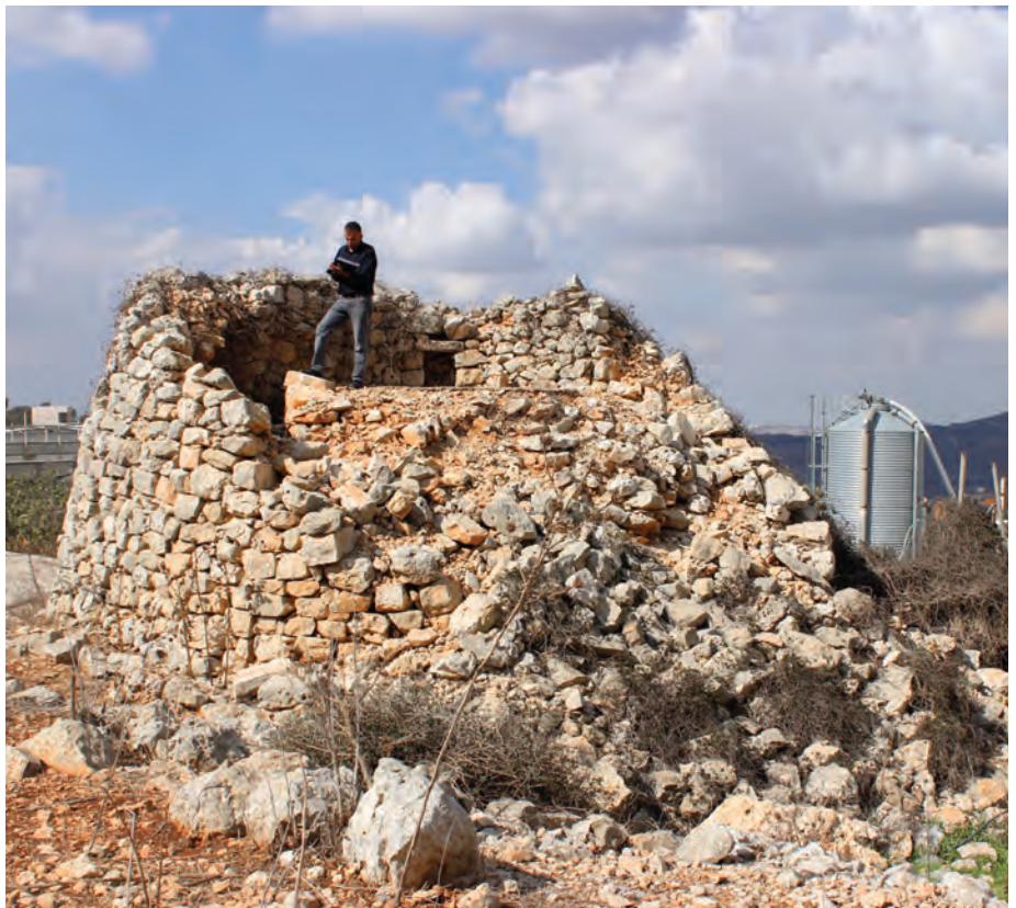
Figure 4. Corbelled, round stone watchtower, looking west, 2016. Photo by S. Al-Houdalieh.
