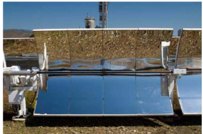
Fig. 2. Photograph of the parabolic trough solar collector (Garcia et al. [38]).
