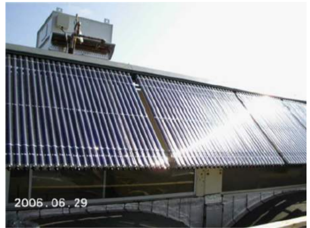
Fig. 6. Photograph of the solar heat pipe vacuum collectors (Bourdoukan et al. [44]).
