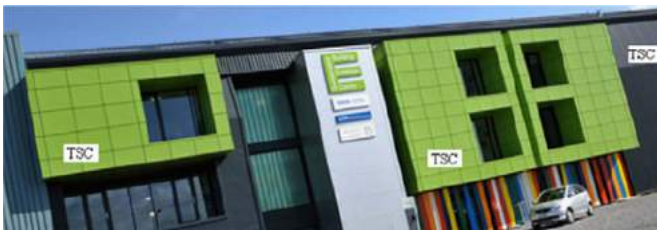
Fig. 10. Photograph of transpired solar collector (Shukla et al. [52]).
