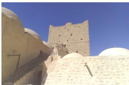
pl. 9. The stairway leads to the keep
