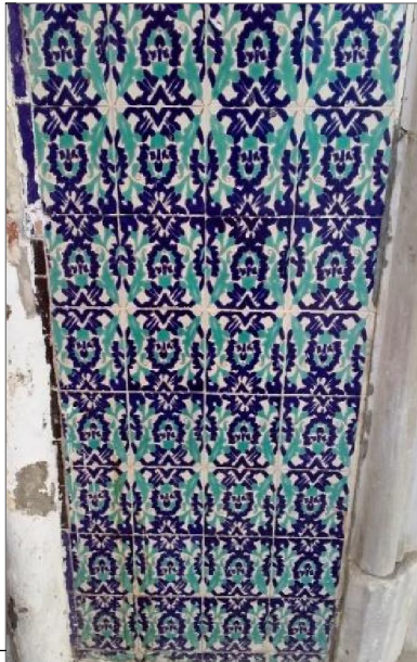
Figure (10) The lower decorative strip that has been replaced (Photo by the researcher)
