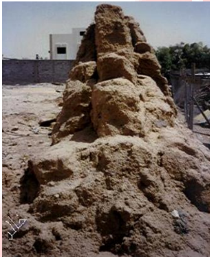
Pl. 6. Sectional of the third fence and its thickness is graded from bottom to top
