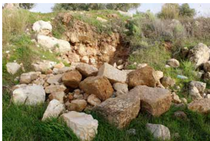
Figure 8. Destruction of the remains of the fortification system at Khirbet el-Lauz (compare with fig. 7), looking east, 2018. Photo by the author.
