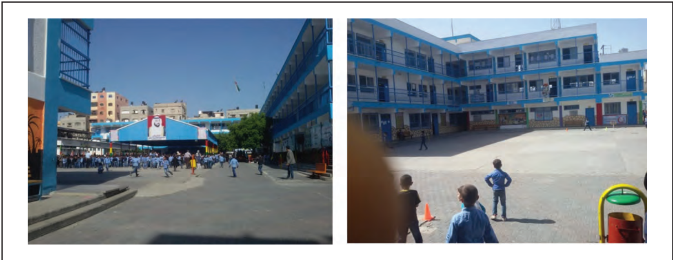
Figure 8. Khalifa Bin Zayed School temporary shelter in the event of war.
